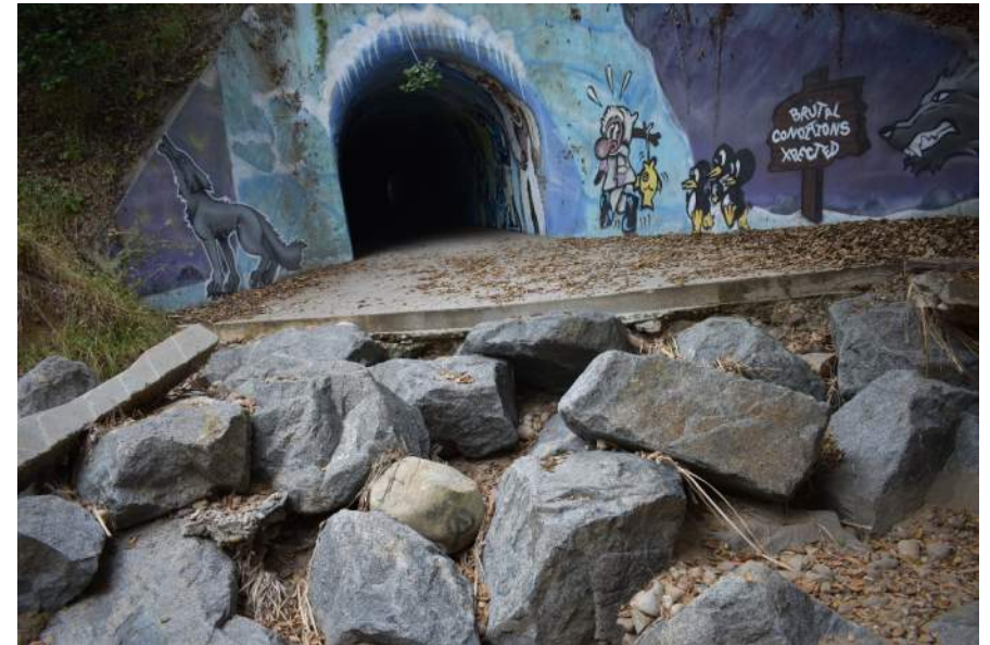
Rock riprap in the foreground at existing arch culvert outfall
