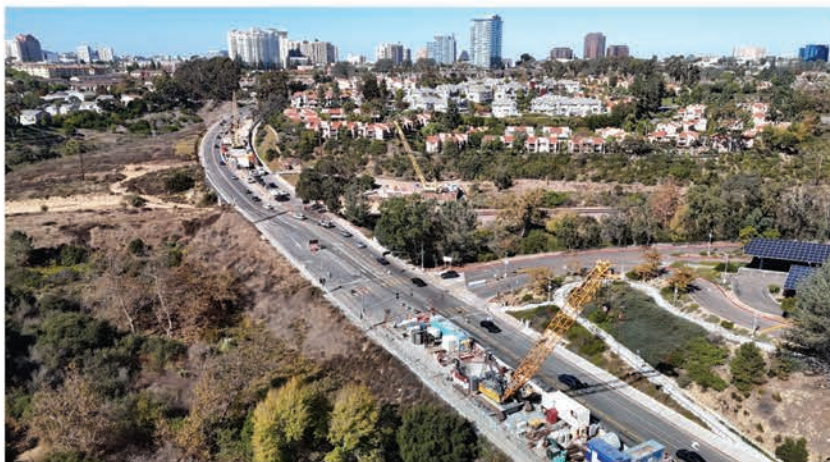
Genesee Avenue work area near UC High School overlooking Rose Canyon.
