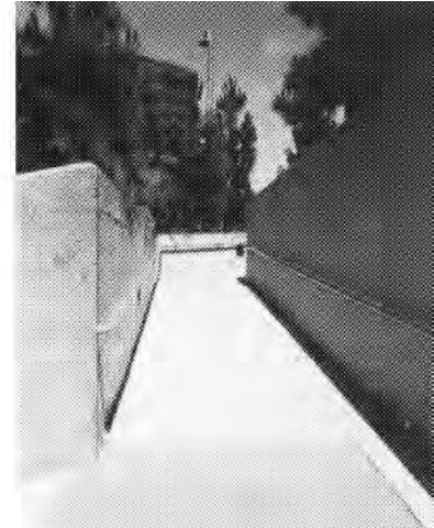
Access to overpass is too enclosed for comfort and safety.
