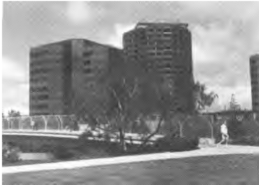
Good example of landing area at the end of a pedestrian overpass.
