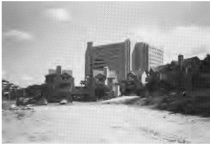
Poor transition between tall structures and adjacent small scale projects.
