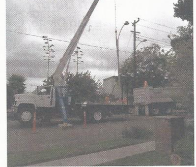
Angell on the west end...power lines getting removed after going underground with utilities.
