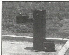
New Drinking Fountain
