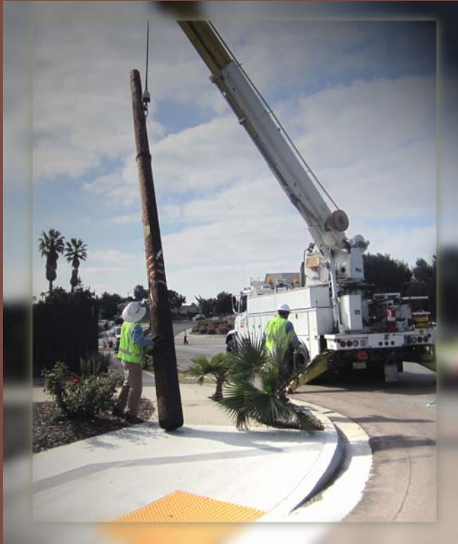
The final pole was removed on Stresemann and Ducommon.
